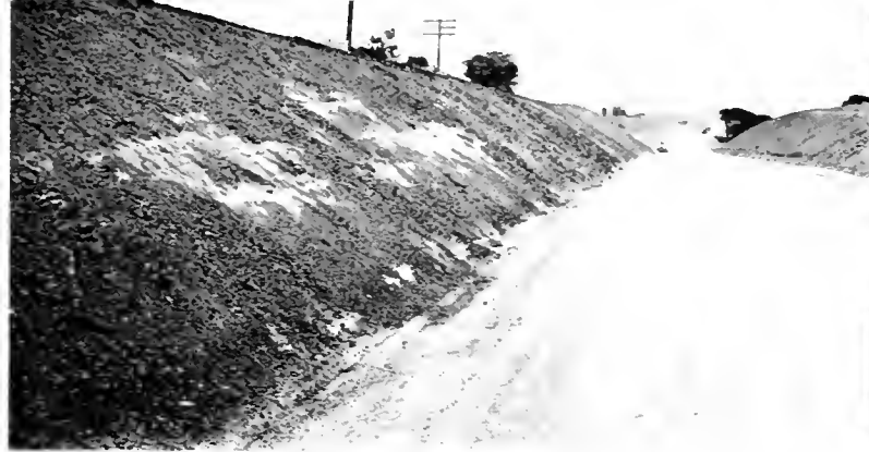
Lumps or granular particles can not be expected to stick to a 1\frac{1}{2} :1 smooth surface. Roughening is necessary
